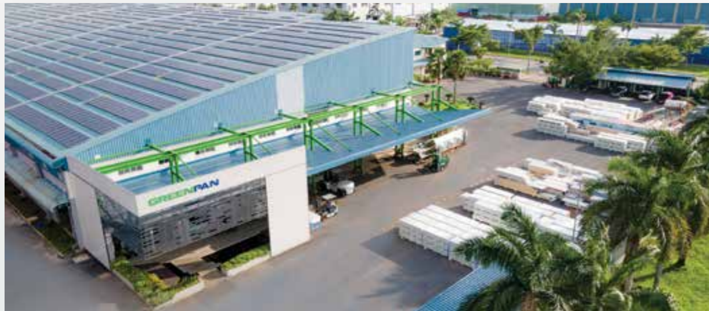
View of the Panel Manufacturing Plant – Greenpan Joint Stock Company at Tan Tao Industrial Park, Binh Tan, Ho Chi Minh City
